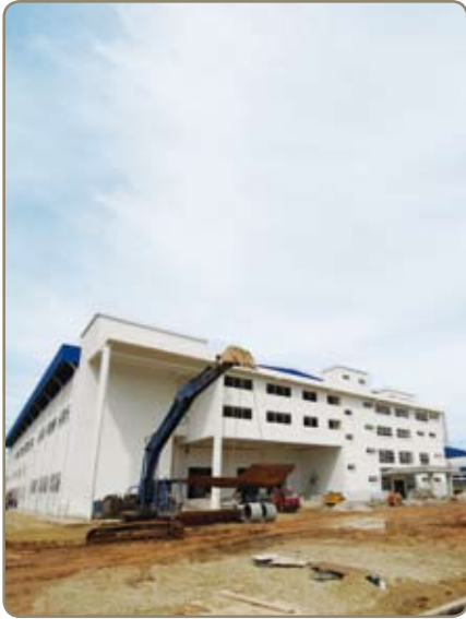
Packaging/Bakery: New factory under construction at Meru, Klang
